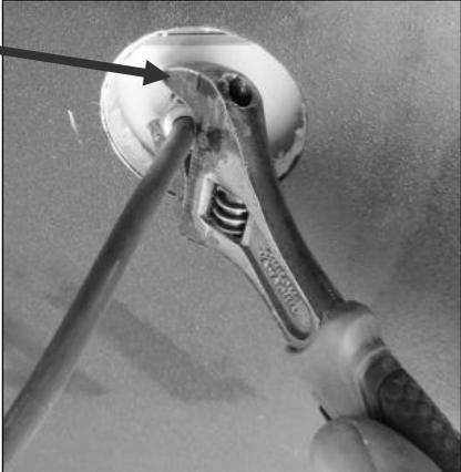
Wrench inside to keep solenoid valve from spinning
